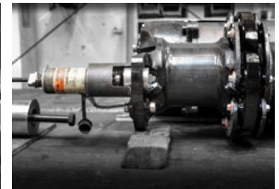
Replacing of spherical bearings
